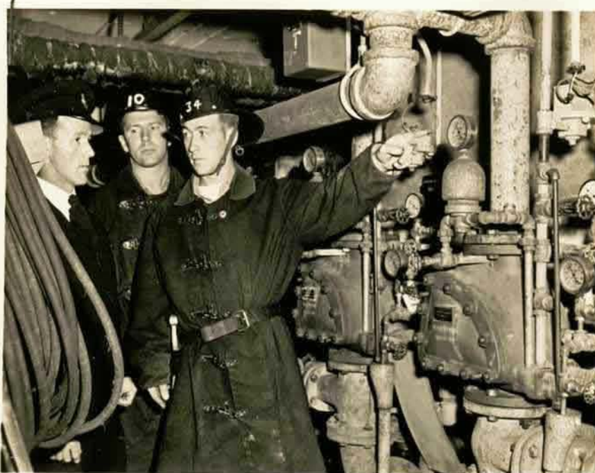
Neg. No. DB 7846 Dispo: L HQ Dest Photo's Manuel Dept. FIRE HALL Dept. FIRE SPRINK- LER SYSTEM IN HMC COMMUNICATION SCHOOL.
