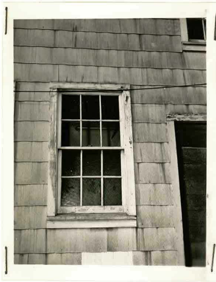
Neg. No DB 8003 Dispo: L HQ Dest [ ] Photo: Arndt E. Dep: HMCS "BRUNSWICK" Cap: CONDITION OF PAINT on outside walls of main building of HMCS "BRUNSWICKER".
