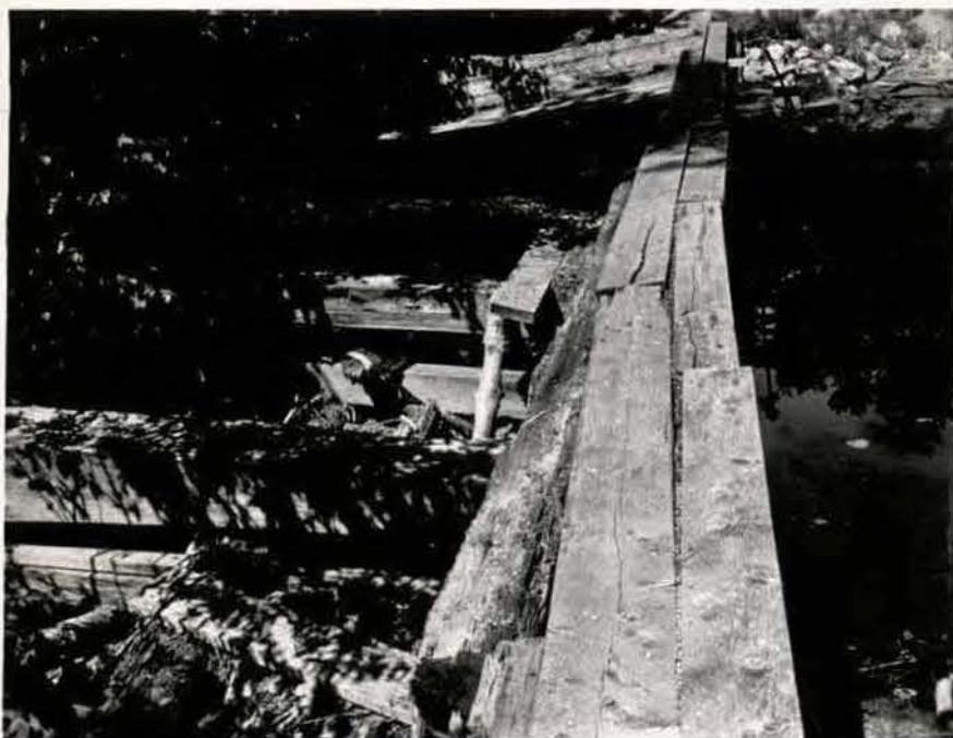
DB 9278 Dispo: L.✓.HQ..Dest.. Photog A ndt . Dept. Maintenance Water Dam at Kadie Lake.
