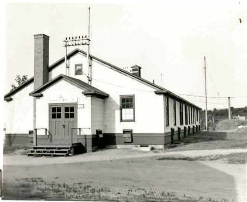
Neg DB 9389 Dispo:L..HQ..Dest.. Photog. Ellis Dept. Fire Shot of bldg. after garbage removed.
