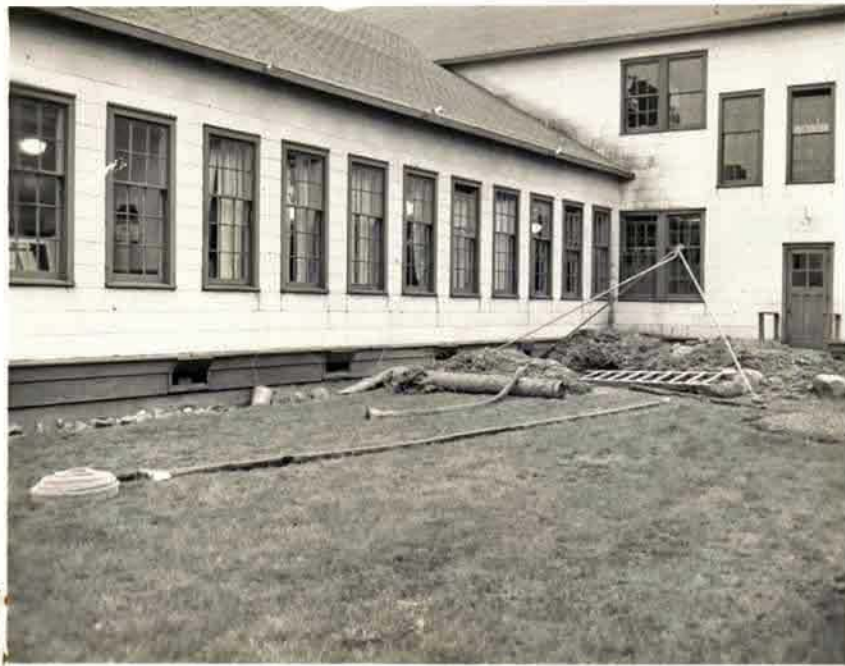
Neg. No. DB 9921 Dispo. L. ✓ HQ. Dest.. Photo 'g. Carroll Dept. Comm. School Caption. Grounds at Comm. School. Litter left by Maintenance when repair to water line.
