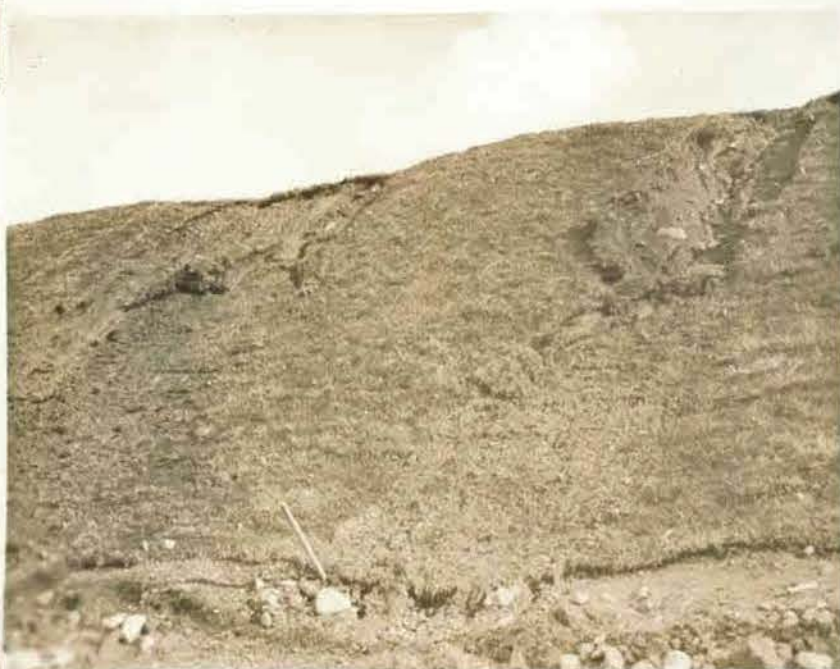
Neg.No. DB 9905 Dispo. L. / HQ. Dest.. Photo'g Manuel Dept. Maintenance Caption. Condition of new soded area on west side of sports field after storm.
