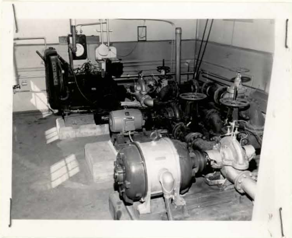
DB 12227 Dispo: L..HQ..Dest.. Photog. Porter Dept. Maintenance New equipment in pump room
