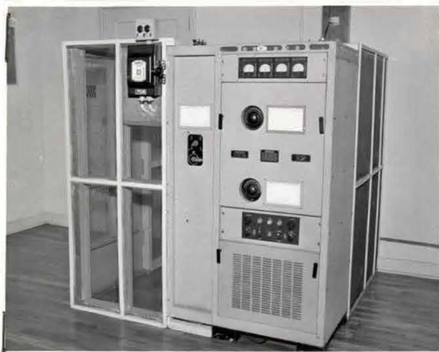
HMCS Cornwallis 12904 L Porter Comm School 27-8-59 Comm. Equipment. PV 500 LM Transmitter.
