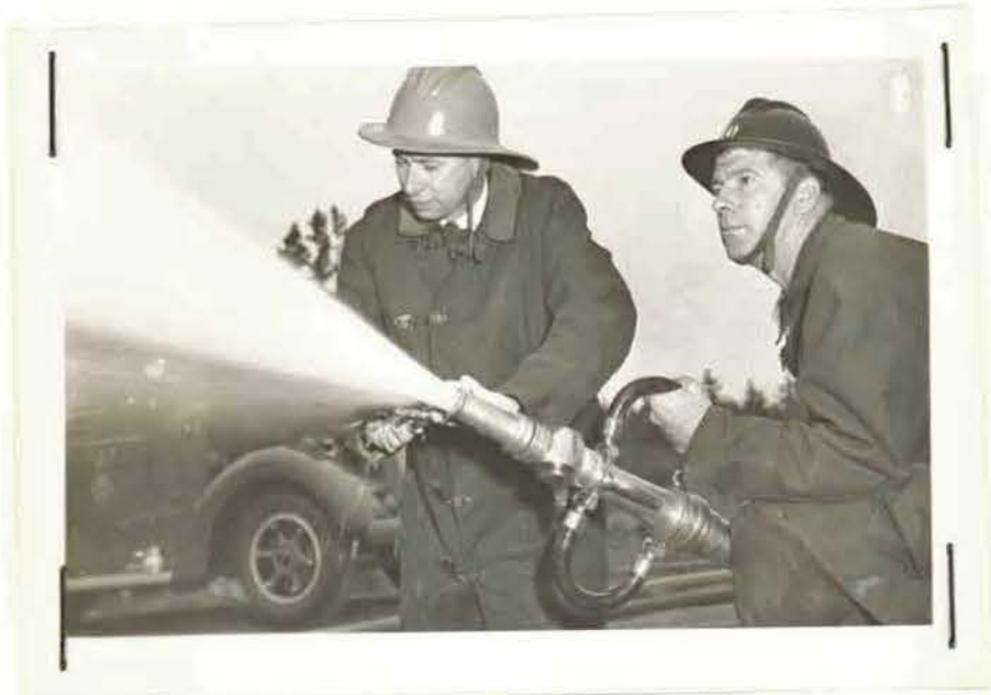
Firemen measuring pressure of stream from hose.
