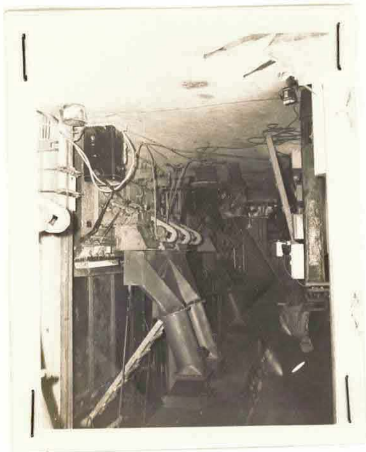
Interior of New Heating Plant showing front of boilers.
