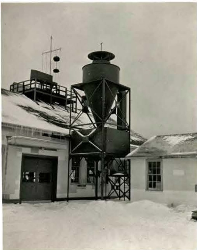
H.M.C.S. CORNWALLIS NEG. NC. DB 19591.... DISPC L x HQ D PHOTCG. Estensen..... DEPT.. Maintenance.... DATE. 25-1-65..... CAPTION. Sawdust disposal unit.
