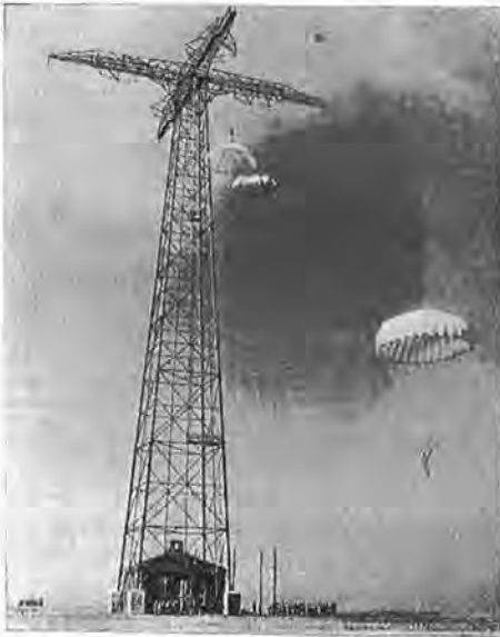
This is the Parachute Jump Tower, Shilo, Man., which is used by PPCLI for parachute training. The tower is 256 feet high with four arms — three free and one controlled. On completion of training from the tower, paratroopers then jump from assault aircraft. A similar tower is under construction at the Joint Air Training School, Rivers, Man.
