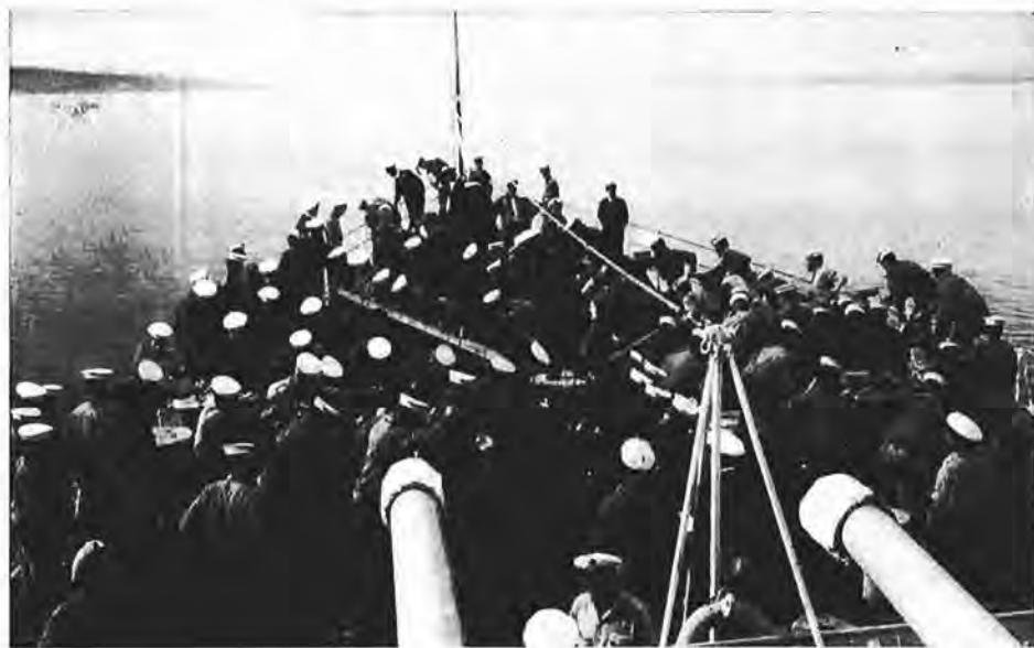
Steam and electricity do the heavy "pushing" in today's warships, but it's necessary, all the same, to know how to employ "handraulic" power in case of damage or breakdowns. So we see men under training in the "Ontario" manning the capstan bars and weighing anchor by hand. The caption accompanying the photo failed to say whether they broke into any sea chanteys. (OC-158-1).
