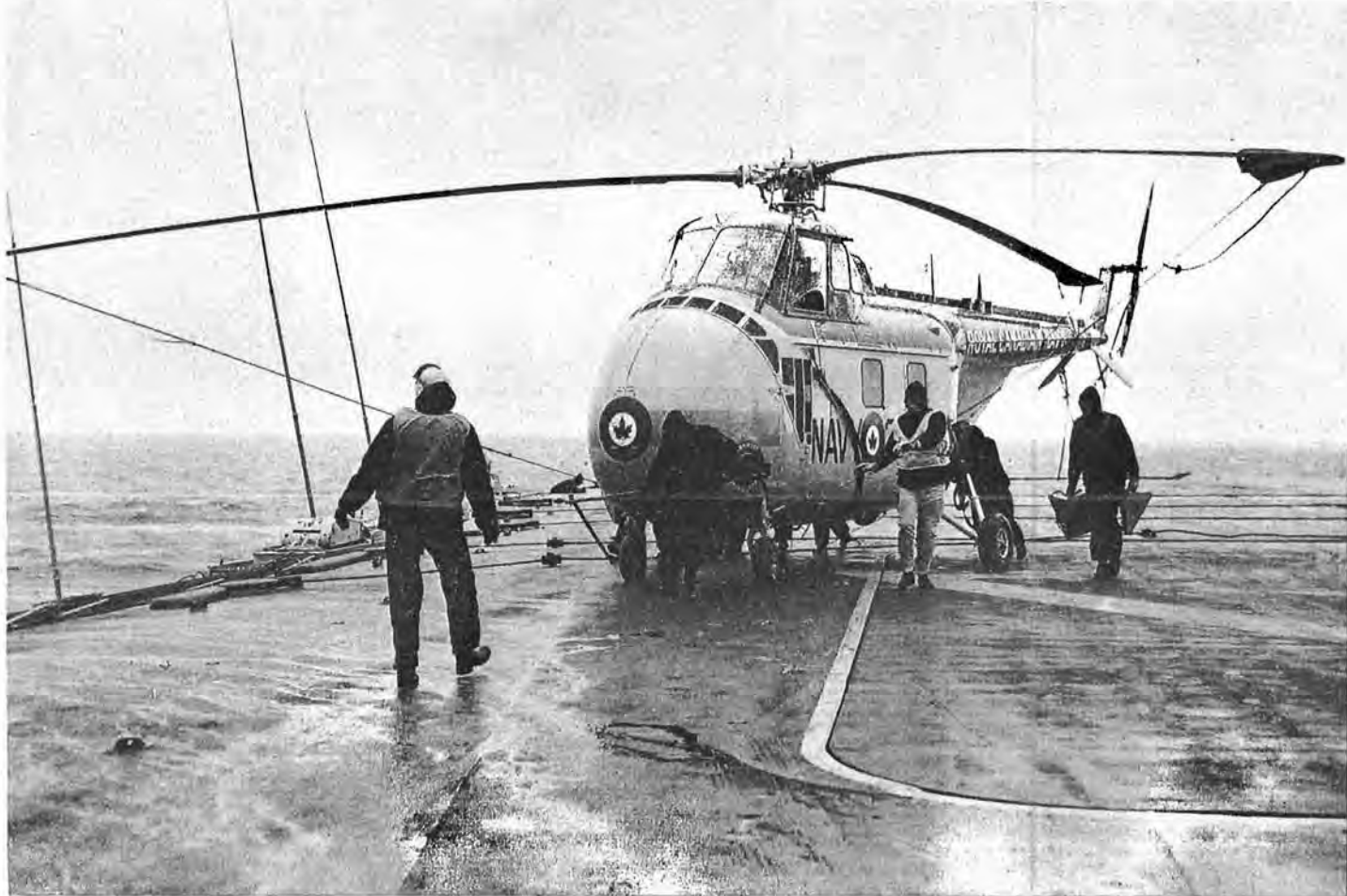
Spray swept from the grey sea by the Arctic wind forms rivulets on the Bonaventure's flight deck as "Pedro", the rescue and utility helicopter is repositioned. The flexible rotor blades are lashed down to keep the motion of the ship from snapping them. The picture was taken during Exercise Traplaine. (HS-66400-108)
