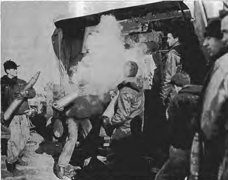
Two more coming up for Red shore batteries at Inchon. (CA-463)
