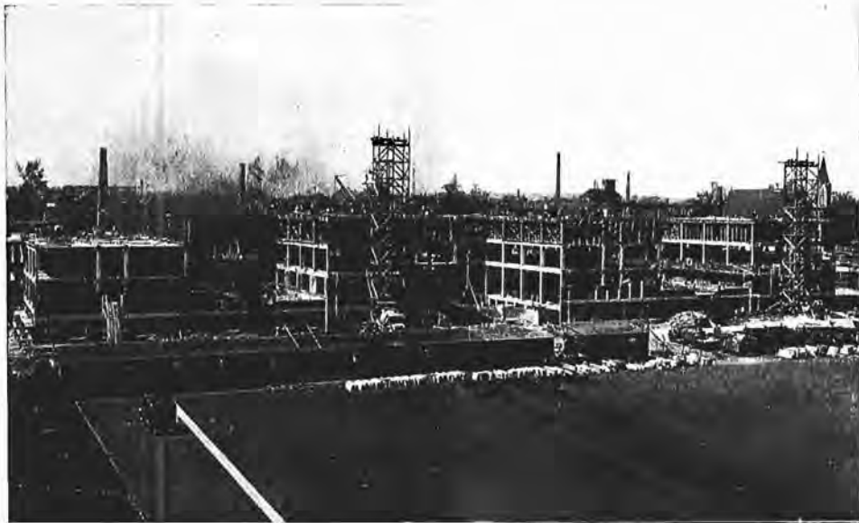
The new men's accommodation building, now under construction at HMCS "Stadacona," Halifax, as it looked in the latter part of May. (HS-11119.)
