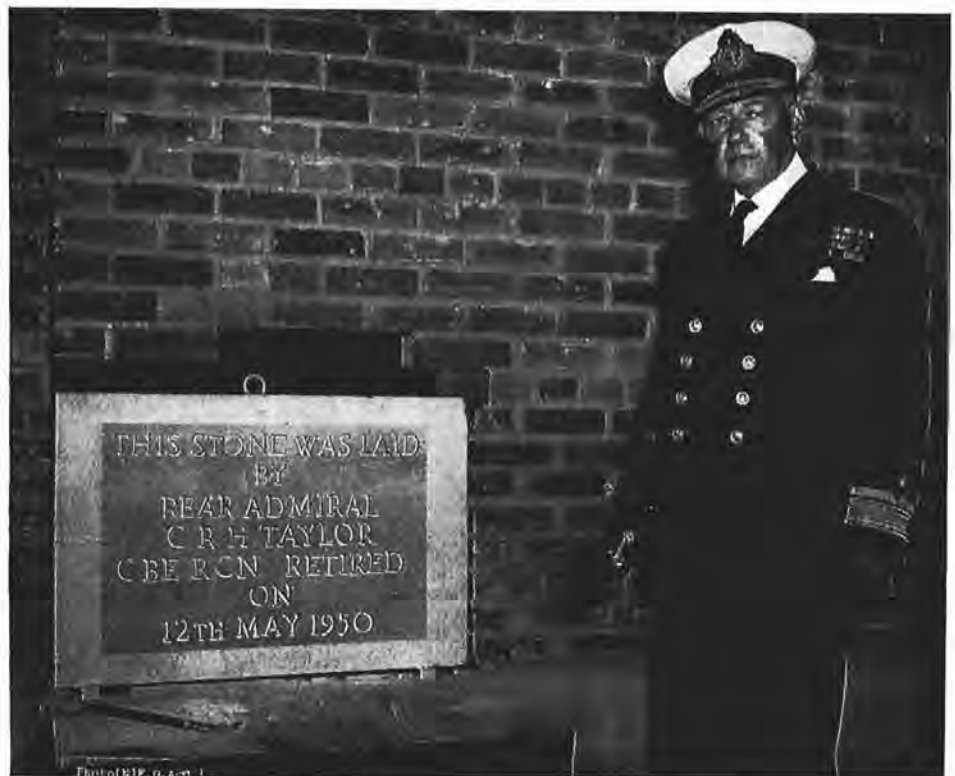
With a tap of his engraved silver trowel, Rear-Admiral C. R. H. Taylor, CBE, RCN, Ret'd., declared the cornerstone of the new "Stadacona" men's accommodation building "well and truly laid." Admiral Taylor campaigned vigorously for the new building during his term of office as Flag Officer Atlantic Coast and it was largely through his efforts that the project was undertaken. (HS-10916.)
