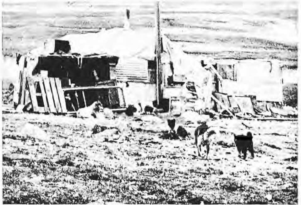
A fine example of modern Eskimo architecture is this Padloping Island bungalow, constructed of canvas, crating, seal skins and even an old bed spring.
