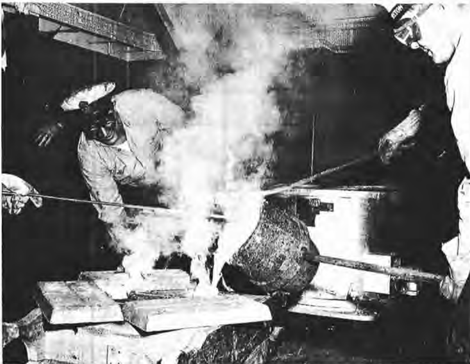
Molten metal hisses into a mould in the foundry on board the Cape Breton , Pacific Command escort maintenance ship. (E-58765)
