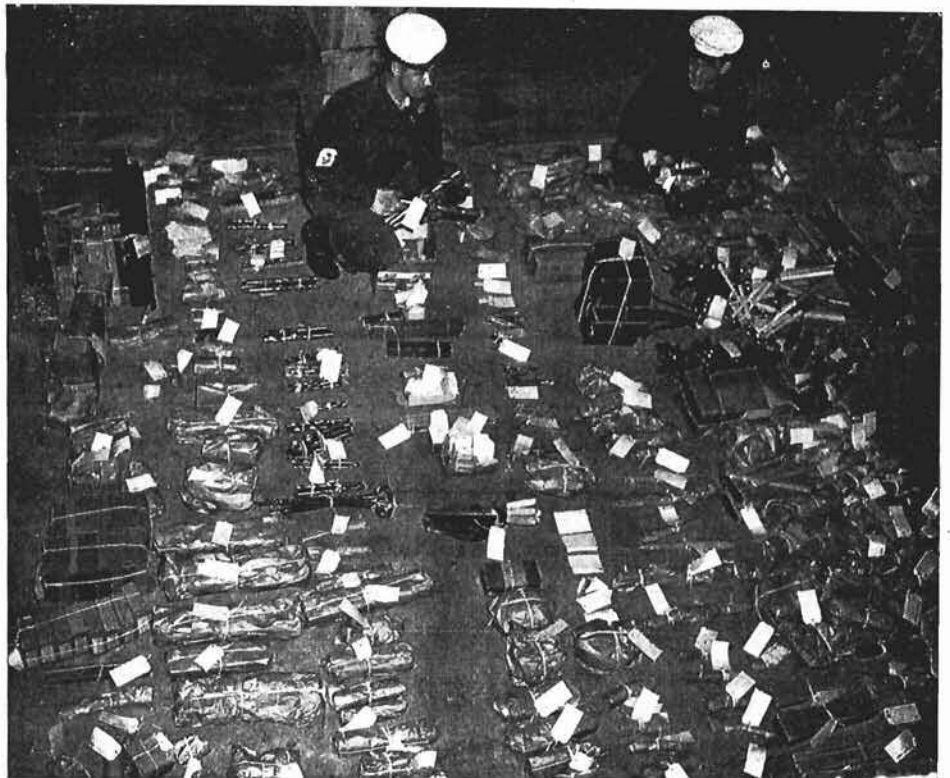
It took more than a refit to make HMCS Quebec ready for sea. Thousands of stores items had to be gathered, checked, tagged and properly stowed before she should be considered ready to operate. Provisions, paint, brushes, cordage, tools, clothing, nuts, bolts, spare parts, light bulbs — those were only a few of the items. Here two members of the advance party, Ordinary Seamen H. Young and G. Gaudon, lay out some of the smaller-sized articles in preparation for their being stored in the ship. (E-16942).
