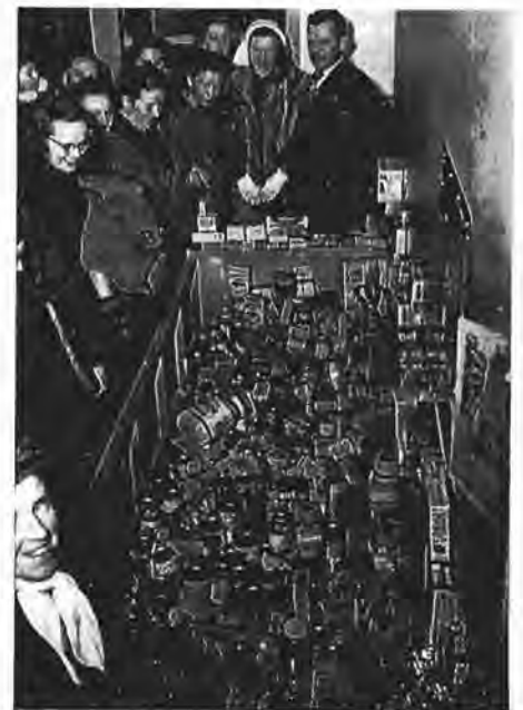
Pictured here are some of the nearly $300 worth of groceries received at the show put on for the benefit of PO and Mrs. George Davies, whose home at Belmont Park was destroyed by fire January 11. The show was held in the John Stubbs Memorial School under the auspices of the Belmont Park Town Council and was organized by PO James Waller. (E-21336).
