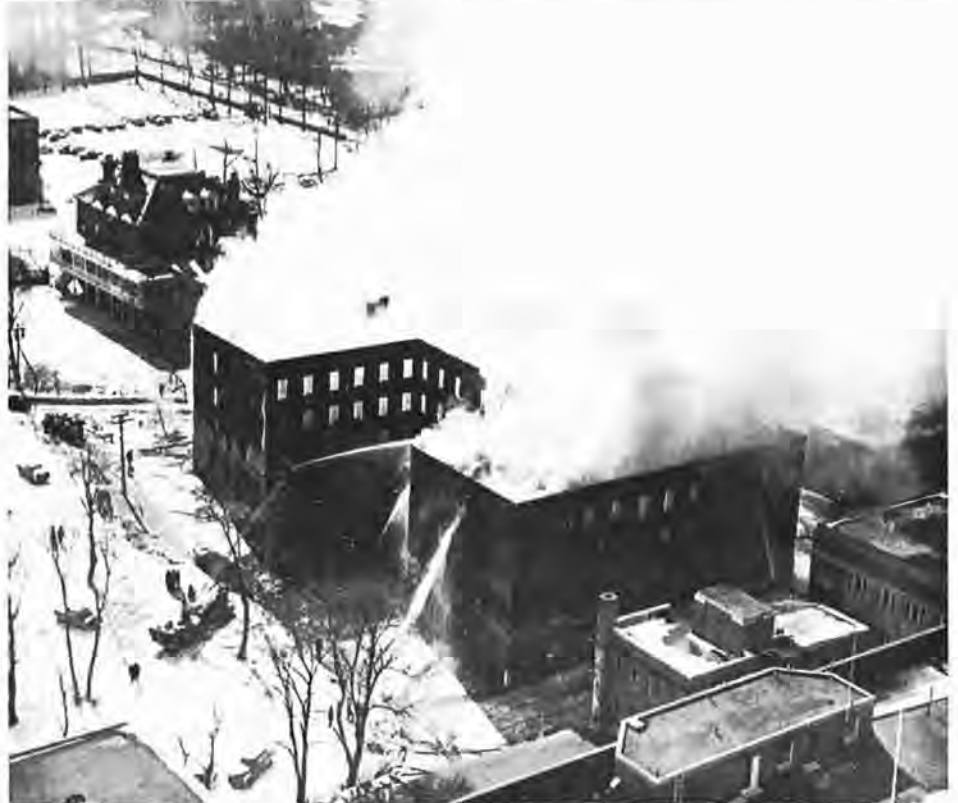
An alert fire sentry (AB Roy Turner) and the discipline of the 127 men in the building won credit for the absence of loss of life when fire which broke out at 3 a.m. destroyed the chief and petty officers' living block at Stadacona on February 27. Residents had to flee so quickly—some of them by sliding down ropes from the third floor—that most of them lost clothing and personal effects. Halifax and naval fire departments kept the flames from spreading to nearby buildings. (HS-22846)
