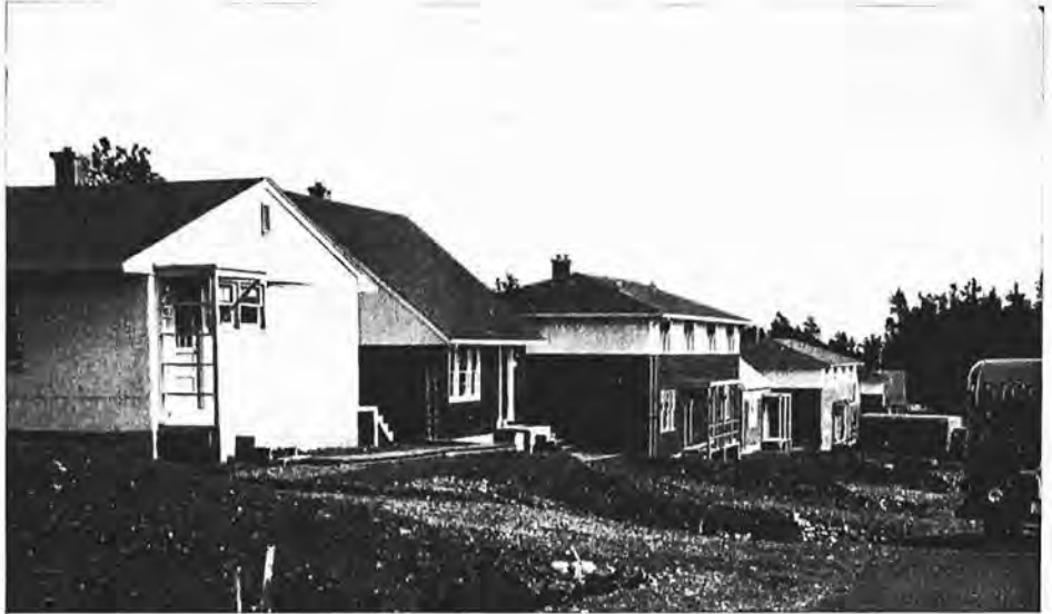
A view of the first houses to be occupied at the new naval married quarters development at Belmont Park, near Royal Roads. (E-13744).
