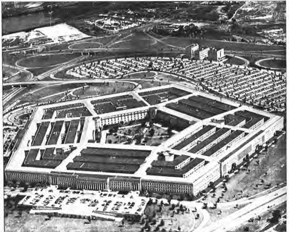
An aerial view of the famous Pentagon. Staff officers at Niagara are said to claim there should be a special distinction for those who become fully conversant with the intricacies of this building, and its approaches, in the course of a normal appointment in Washington. (U.S. Army photo).
