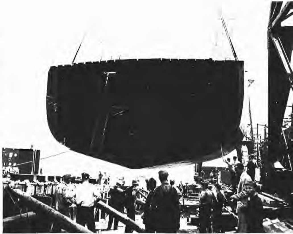
Laying a keel in this day is accomplished by a method much different than that of yesteryear. The first section of the destroyer escort which will one day bear the name HMCS "Chaudière" is shown as it was lowered into place immediately after the launching of HMCS "Saguenay" at Halifax shipyards.
