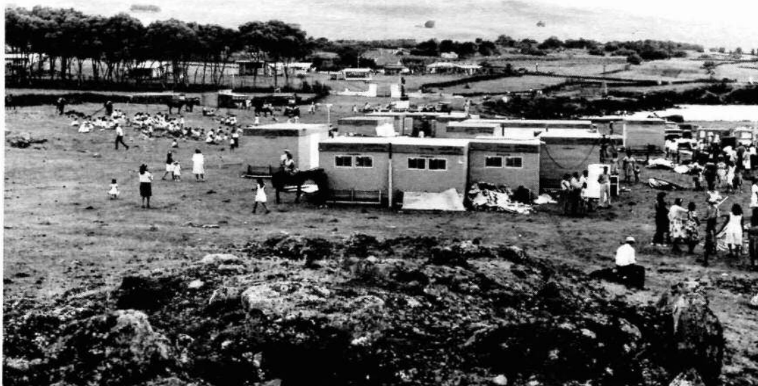
RAPA NUI HILTON under construction. Photo: Canadian Department of National Defence
