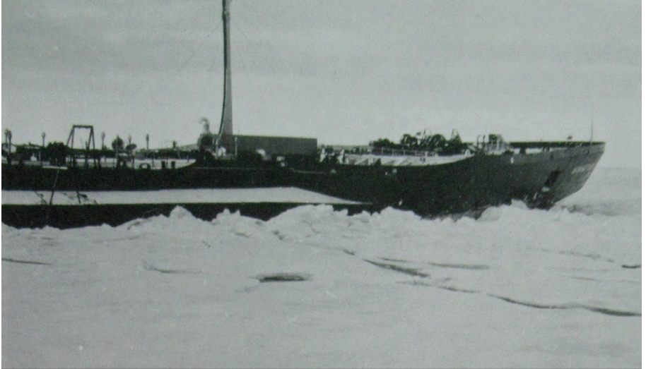
Figure 3-10: MANHATTAN's bow at rest in a ridge.
