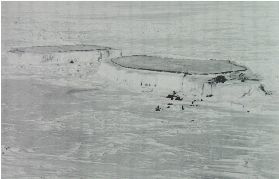
Figure 2-1: Two ice islands grounded north of Prudhoe Bay. Attempts were made to fix these to the bottom in order to provide deep water loading facilities for North Slope Alaska oil.
