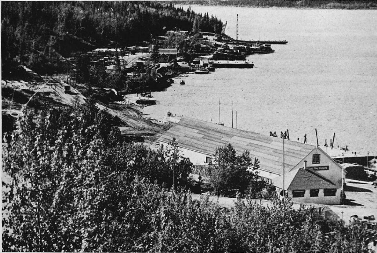
Section of loading facilities at Fort Smith, northend of the 16-mile portage from Fitzgerald around impassable Pellican Rapids.
