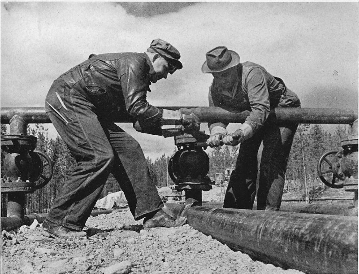
Above:—Soon black gold will be flowing through these pipes. Tightening a valve head.
