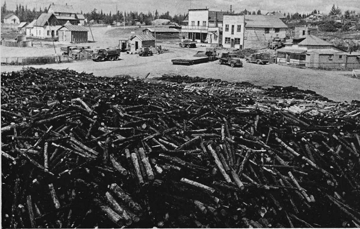
From a stockpile of firewood, photo shows an outpost of Fitzgerald, head of portage on Slave River. Hundreds of trucks and caterpillars are used to transport supplies, equipment, boats and barges along 16-mile overland route to Fort Smith.
