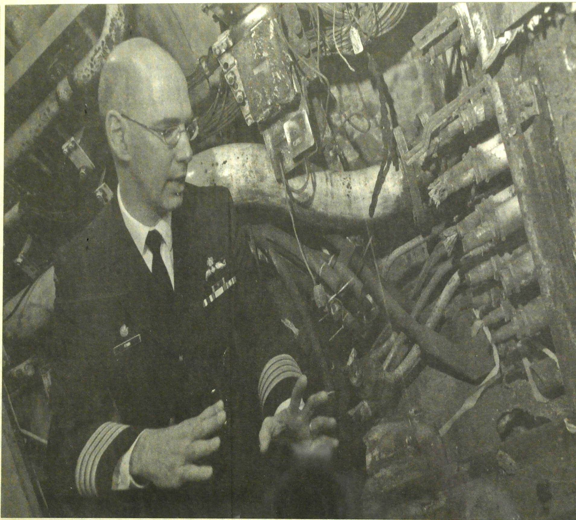
Capt. Pat Finn, senior member of the board of inquiry into the flooding and fire on the Victoria-class submarine HMCS Chicoutimi, shows the damage inside the captain's quarters in this file photo from May. (TIM KROCHAK / Staff)
