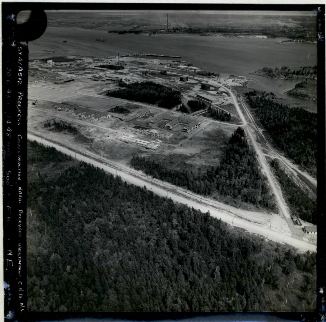
SY.4/A512 20-6-43 500' F.24(SG) Contact Progress Construction, Naval Dockyard, Westmount, Cape Breton Is. Looking NE F.5 In. 1448 Hrs.
