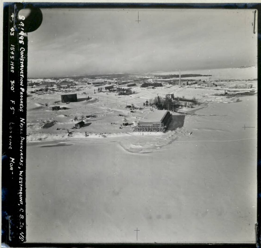
S.4/995 4-2-43 300' F.24(SG) Contact. Construction Progress, Naval Dockyards, Westmount, Cape Breton Is. N.S. Looking N. 1545 Hrs. F. 5 In.
