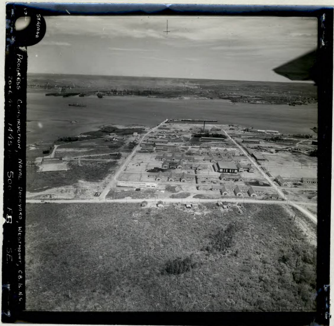
SY.4/A511 20-6-43 500' F.24(SG) Contact Progress Construction, Naval Dockyard, Westmount, Cape Breton Is. N.S. Looking SE F.5 In. 1445 Hrs.
