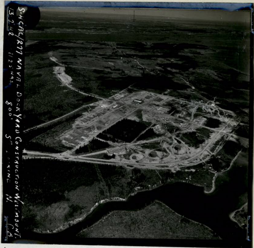
S4CAC/277 13.7.42 800' F.24(C) Contact. Naval Dockyard construction, Westmount, Cape Breton Is. N.S. 1125Hrs. F/5". North.
