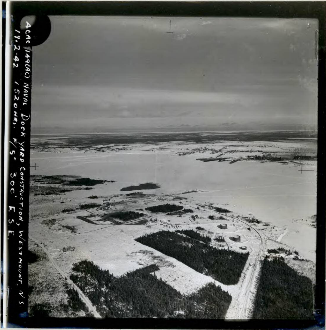
S-149(AC) 19.2.42 300' F. 24 (C) Contact Naval Dock Yard Construction, Westmount, Cape Breton, N.S. 1520 hrs F/5 in. E.S.E.
