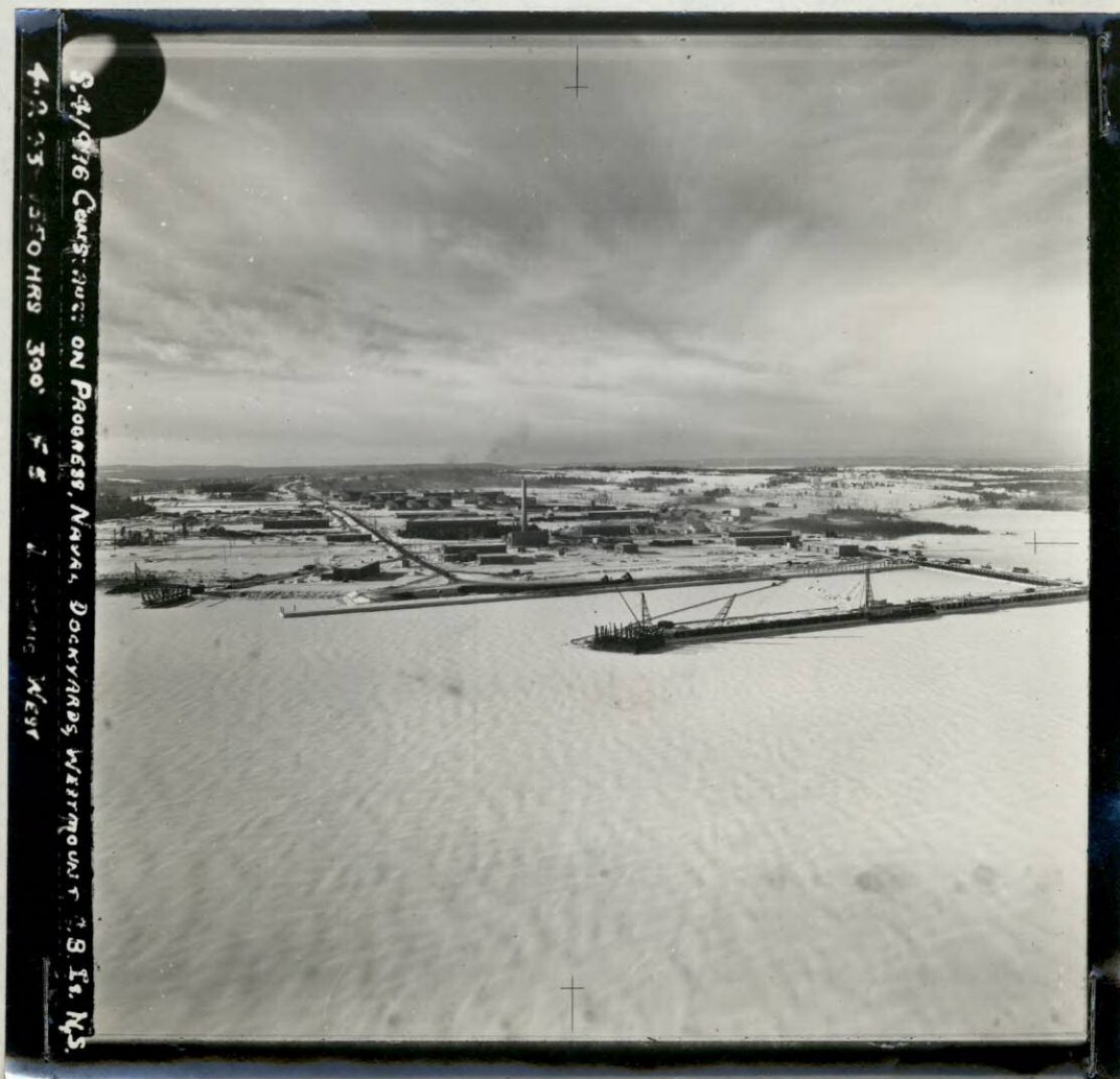
S.4/996 4-2-43 300' F.24(SG) Contact. Construction Progress, Naval Dockyards, Westmount, Cape Breton Is. N.S. Looking W. 1550 Hrs. F. 5 In.
