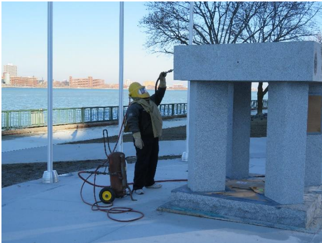
New badges sandblasted onto east and west monument faces and monument cleaned by sandblasting.
