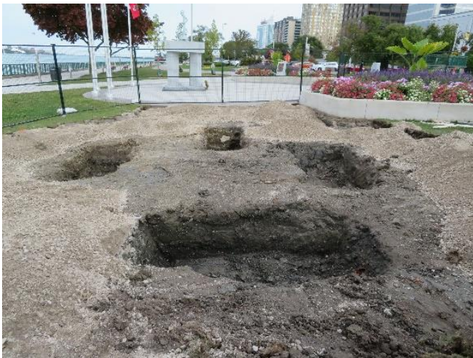
Footing excavations
