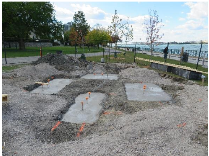
Concrete footings poured.
