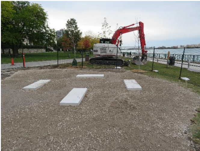
Plaza area back filled & compacted
