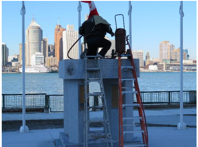
New badges sandblasted onto east and west monument faces and monument cleaned by sandblasting.
