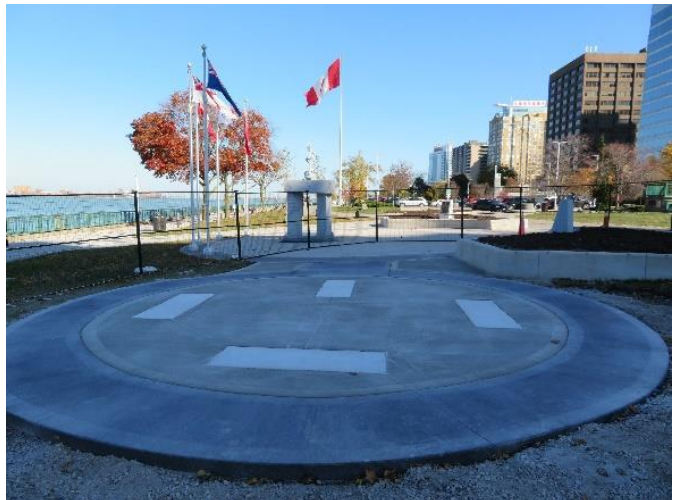
Plaza concrete poured and finished.
