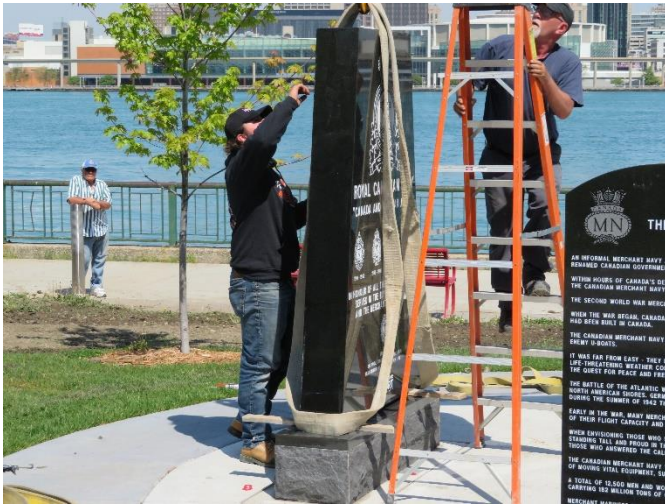
Main Panel level adjustments (left). Panels installed at end of first day (right).
