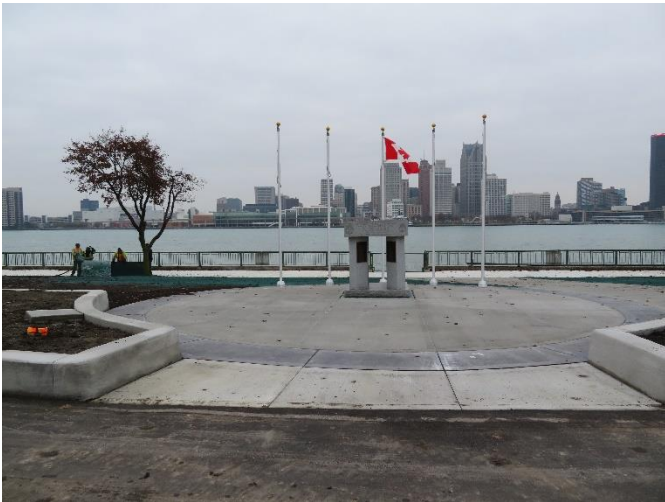
Five new flag poles installed.
