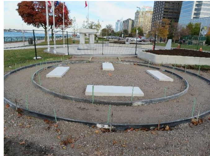
Plaza framed for dual colour concrete design.
