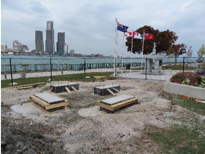
Support bases framed & concrete poured
