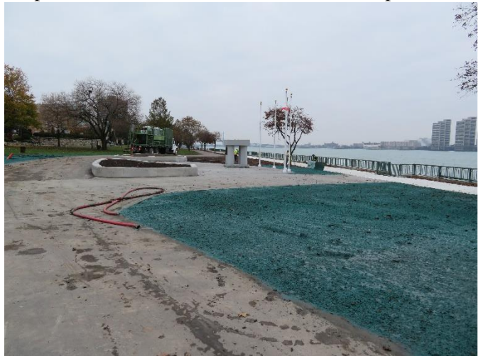
Grass planting in progress.
