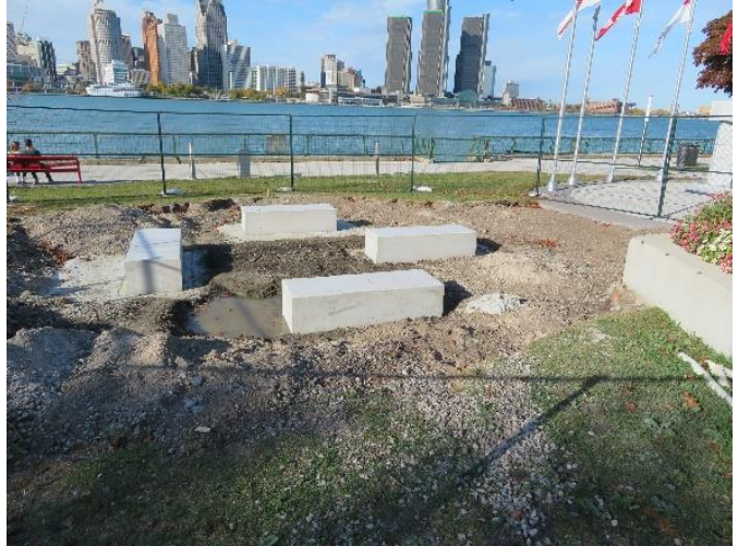
Support bases with framing removed.
