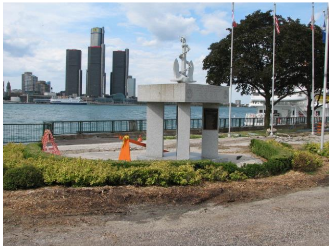
Paving stones and landscaping being removed.
