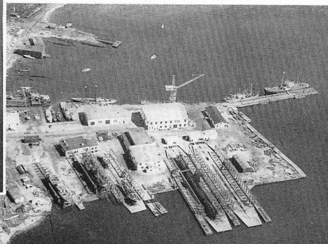
↓ Aerial View of Dartmouth Marine Slips.
